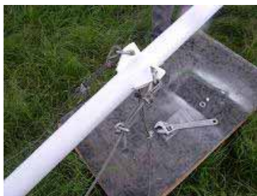
Fig.3.5 Fix wires and clamp
