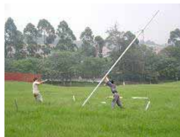
Fig.3.7 Pull to rise tower
