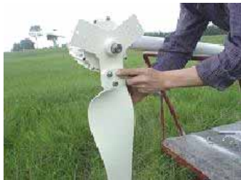
Fig.4.4 Fix wind turbine rotor blade
