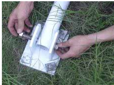
Fig.3.3 Fix tower bolt
