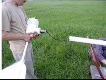
Fig.4.1 Drill through the tower tube to the electric wire
