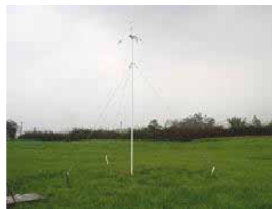
Fig.4.7 Completing the wind turbine system installs
