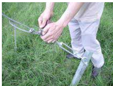
Fig.3.6 Fix malleable clamp
