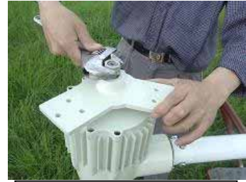
Fig.4.3 Fix wind turbine rotor hub
