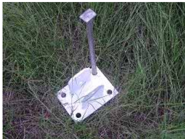
Fig.3.2 Fix tower base
